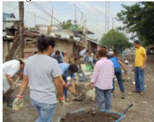
Pitching in to give Rosa's house a new floor
